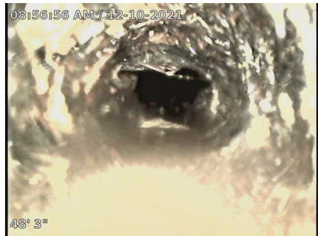
Interior of Pipe
