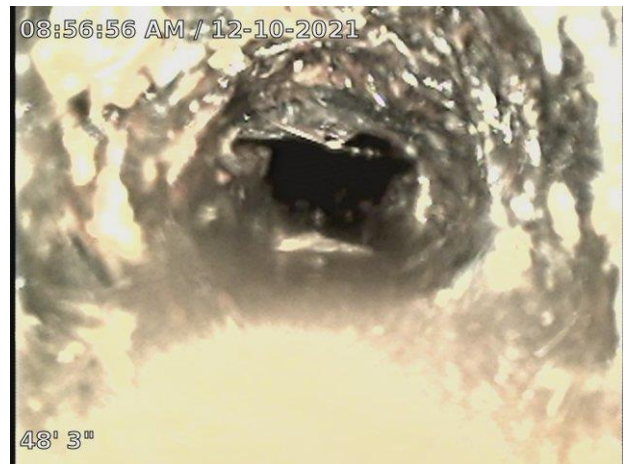
Interior of Pipe
