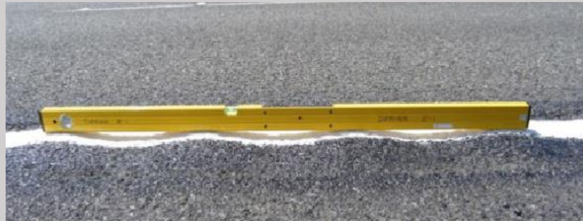
Figure 2. Sinusoidal Rumble Strip - Longitudinal Section
