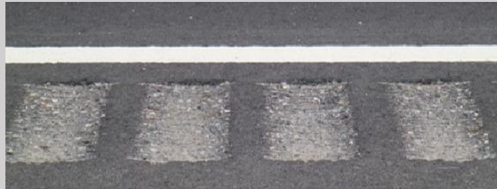
Figure 1. Rectangular Corrugated Rumble Strip – Longitudinal Section
