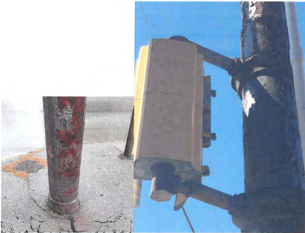
One of two main signal support poles. Hollow steel, both are ancient and badly corroded. One is missing its protective top cap, resulting in exposure to rain, snow and wildlife Typical fixture attached to steel pole. Severe corrosion all around, including the near amputation of the fixture's bottom connector
