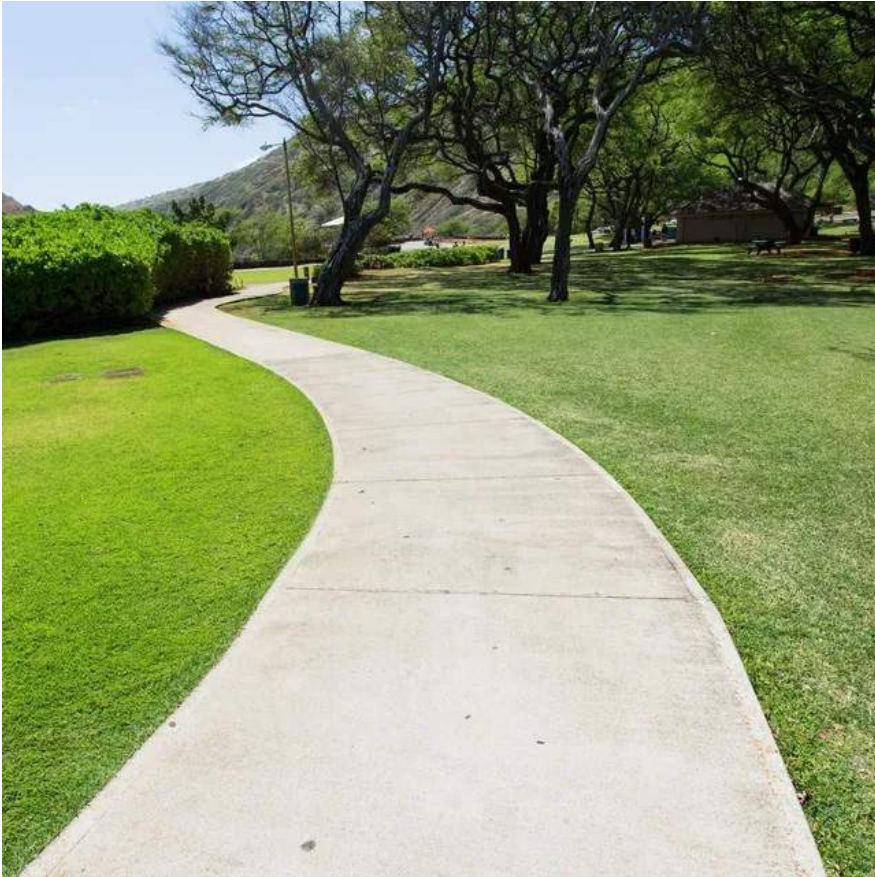
STANDARD CONCRETE (BROOM FINISH AND/OR EXPOSED AGGREGATE)
